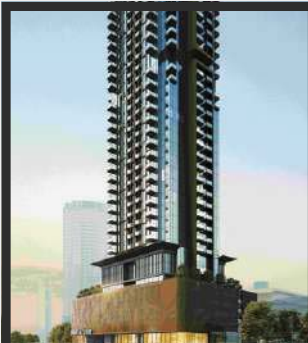
Seslia Tower JVT, Dubai
