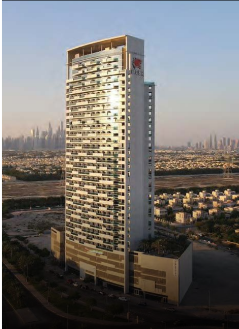
Al Jawahara Tower JVT, Dubai
