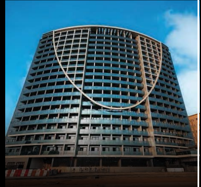
The V Tower Dubai Land
