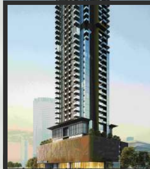
Seslia Tower JVT, Dubai
